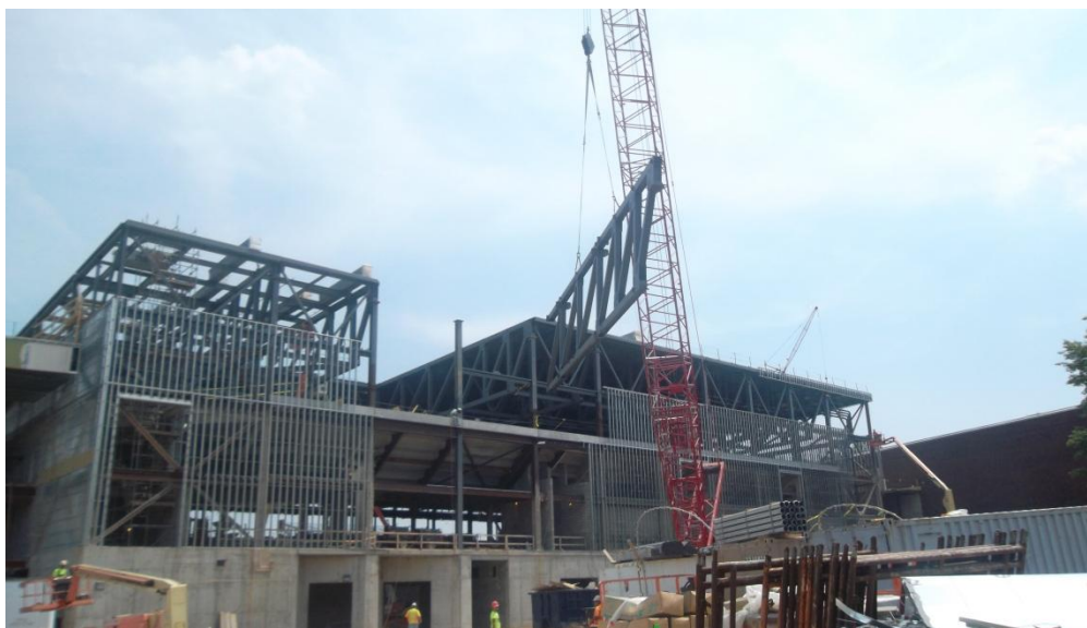
Figure 7. Final truss section erection, taken by Derek Stoecklein
