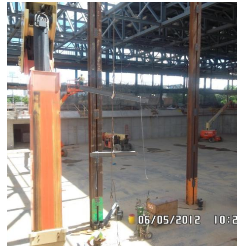
Figure 6. Shoring Towers, taken by Derek Stoecklein
