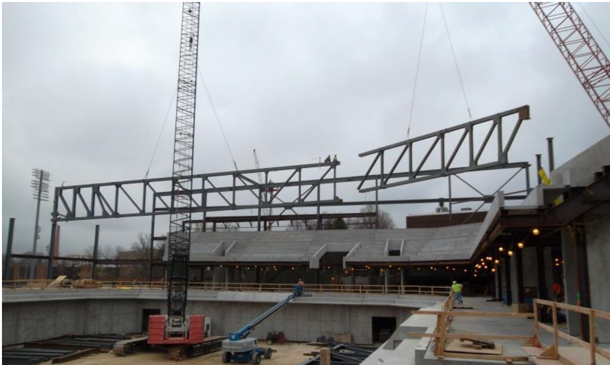
Figure 4. Truss erection image, taken by Ryan Simmons of Gilbane
